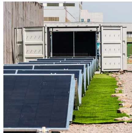
madagascar green energy storage system construction project
